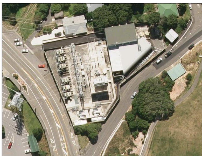
Figure 11-1 Central Park Substation
