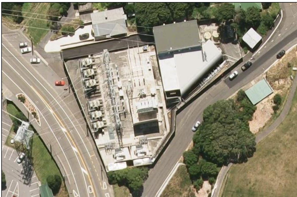
Figure 12-1 Central Park Substation
